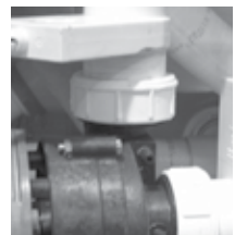
Slice Valve and Pump Union
