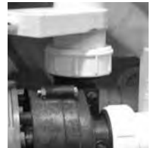
Slice Valve and Pump Union
