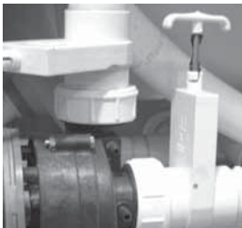
Slice Valve and Pump Union
