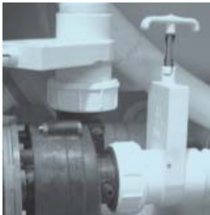
Slice Valve and Pump Union
