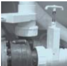
Slice Valve and Pump Union
