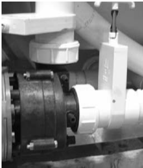
Slice Valve and Pump Union
