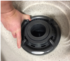
Twist Lock Ring Counterclockwise to Remove Floater
