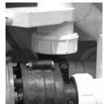
Slice Valve and Pump Union
