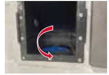
Turn Filter Counter-clockwise to Remove
