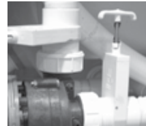
Slice Valve and Pump Union
