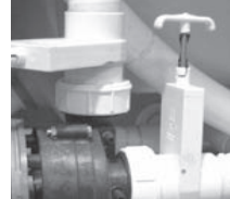
Slice Valve and Pump Union
